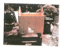
Square up building and cut galvanized welded wire to fit on reinforcement along edges and nail in with fence staples.
